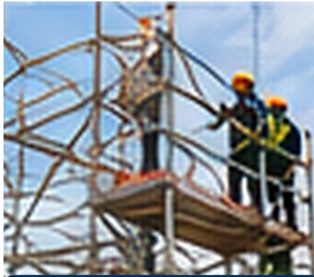
Scaffolding Erection & Dismantling Training
